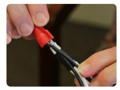
Locate dark grey wire at back of timer and lay it flush with striped ends of white wire bundle. Replace wire nut by screwing clockwise with downward pressure. **Note: make sure wires are snug and cap is secured tightly.**
