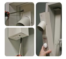
Begin removing electrical raceway from unit by removing small screws at the top and bottom of raceway with a flathead screwdriver. Gently pull raceway out of unit, being careful of wires that are still connected.
